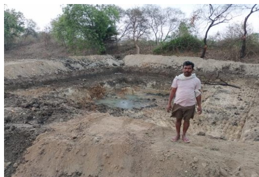
Farm pond under construction
